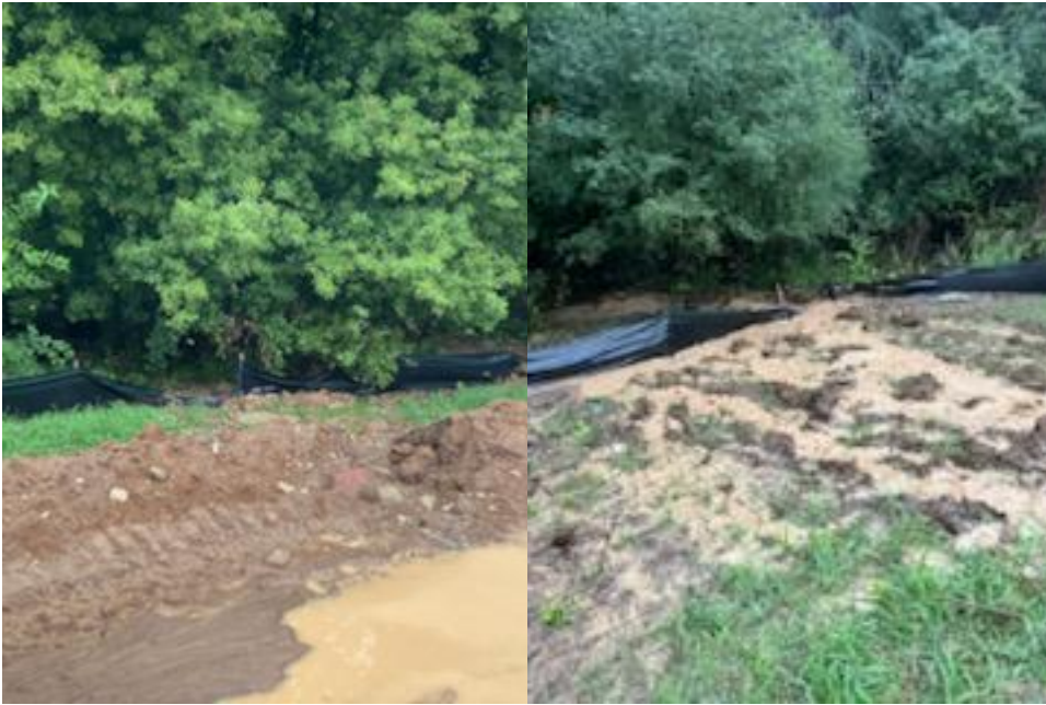
North West corner
