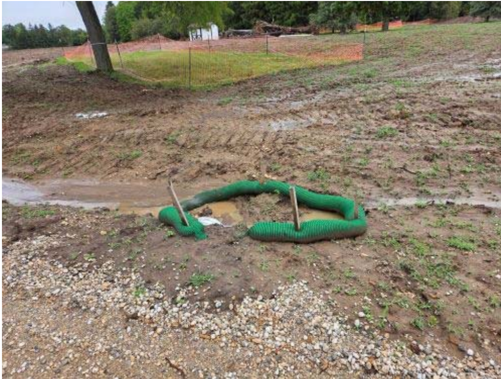
Clean ditch checks
